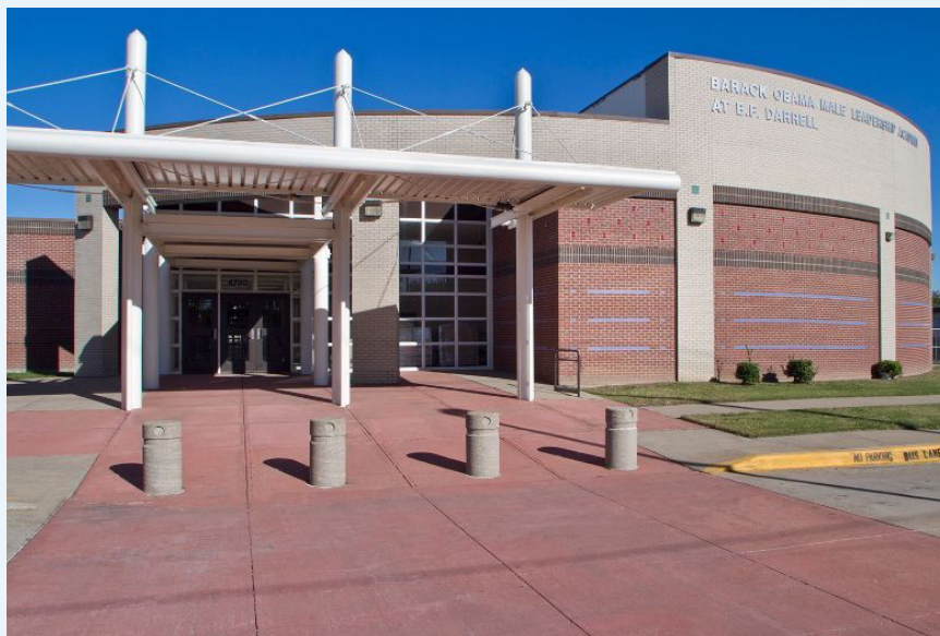
New Tech High School at B.F. Darrell in Dallas Independent School District
